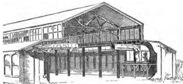
Fig. 6. One-story Building, — Single Fan.
